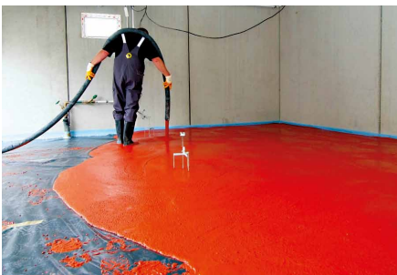
Pouring the screed
